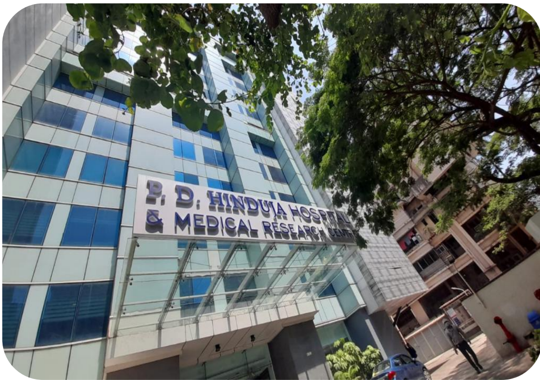
P. D. Hinduja Hospital, Khar
